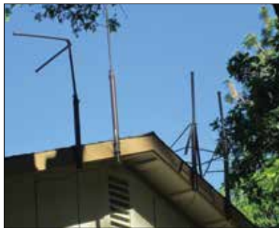
Camouflaged antennas on the roof of the RST Engineering lab.
