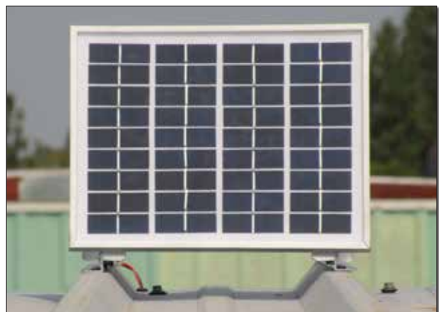
The array mounted on the metal roof (left). Note that there is a rubber grommet where the wires go through the roof into the hangar. The front side of the array as seen from the back wall of the hangar (right).
